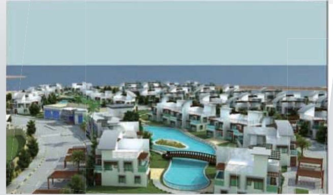
Aerial View (Waterfront Villas)
