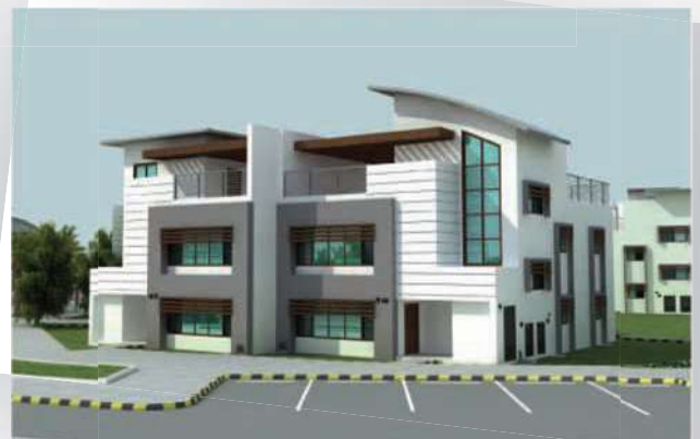
Villa Front View (Waterfront Villas)
